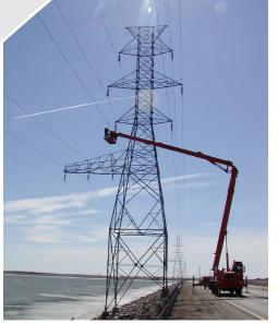
BSI monitors can be installed on energized lines, and will operate in all weather conditions. Research using the BSI demonstrated that it is as reliable as human observers for detecting collisions, and offers the advantage of providing continuous data recording even in the remotest locations. Data retrieval and changes to BSI settings can be performed remotely.
